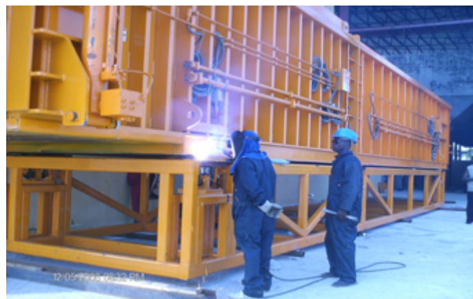
FIGURE 19 PICTURE OF LAWMA MAINTENANCE SECTION
