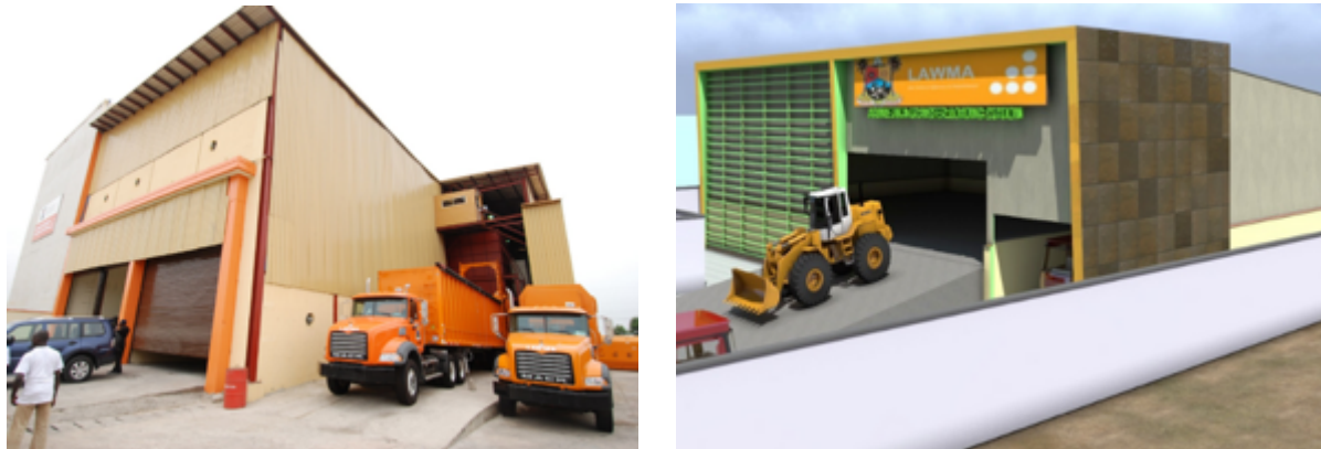
FIGURE 5 IMAGES OF A TRANSFER LOADING STATION IN LAGOS
